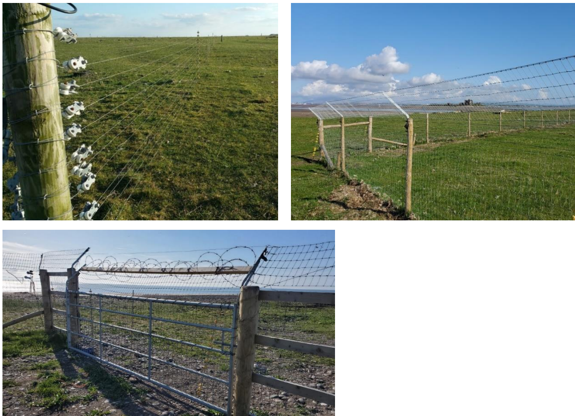
Figure 4: Clockwise from top-left: 12-strand temporary electric fencing used from 2011 to 2020; fence in 2022 showing overhang; gate configuration in 2022.
